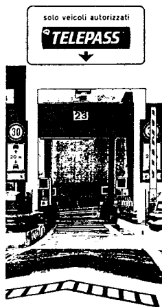
Figure 1: TELEPASS toll station installations (Courtesy of autostrade S.p.A.)
